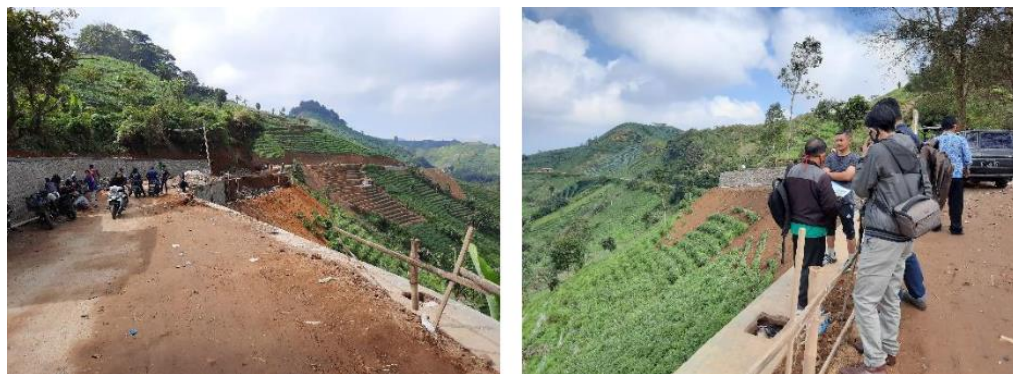
Figure 8. Documentation Of Road Widening
