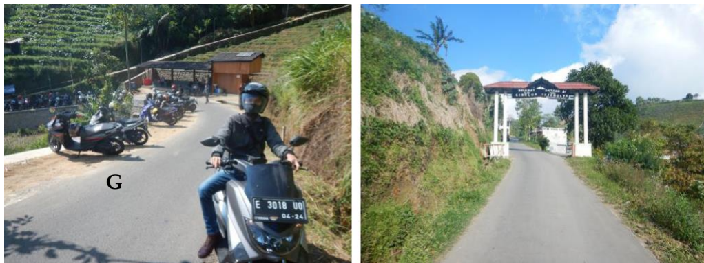
Figure 9. Infrastructure of Panyaweuyan Terraced Area
